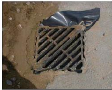
Protected Drain using Visqueen
