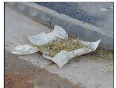
Protected Drain using Straw
