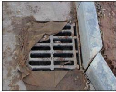
Protected Drain using Terram
